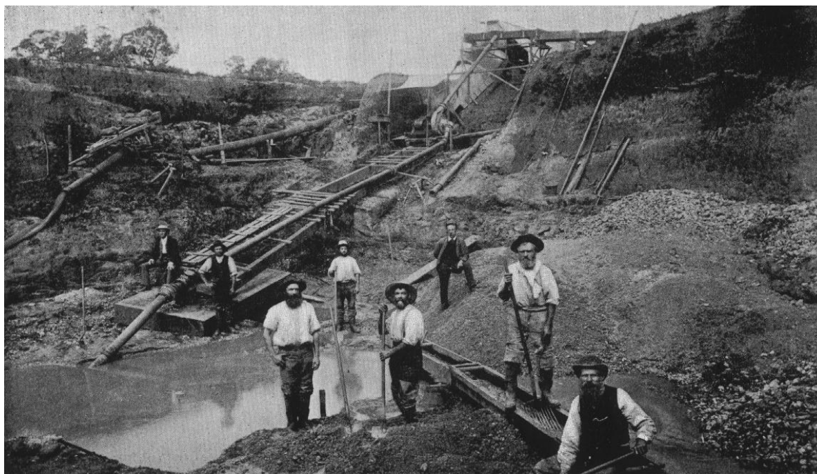
GOLD MINING AT TUMBARUMBA CREEK, N.S.W. (Centrifugal Elevating Pump and Suction-pipe.)
