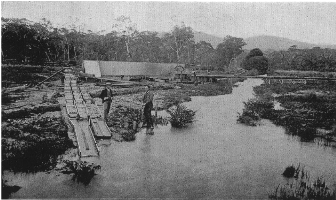
GOLD MINING AT TUMBARUMBA CREEK, N.S.W. (View showing Sluice-boxes, and Pelton Wheel operating Pump.)
